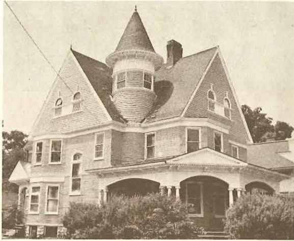
5. THE PALEY HOUSE 802 Park Avenue
