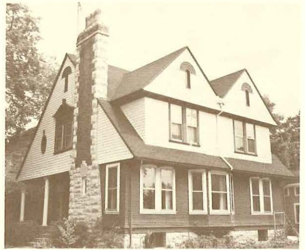
8. THE HOLDEN HOUSE 905 Church Street
